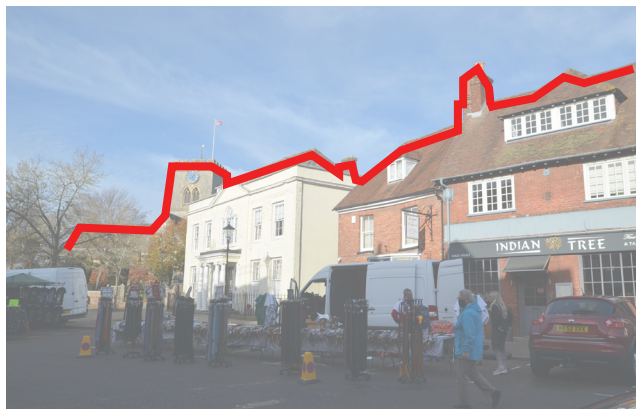
Varied roofscape in Market Pl looking north-west.
