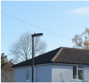
Hipped roof with black pantiles
