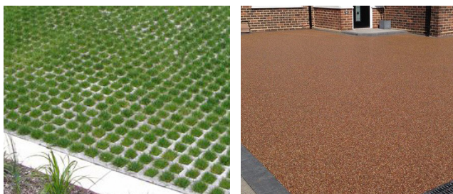
Figure 77: Examples of permeable paving that can be used in the front and rear gardens of residential buildings.
