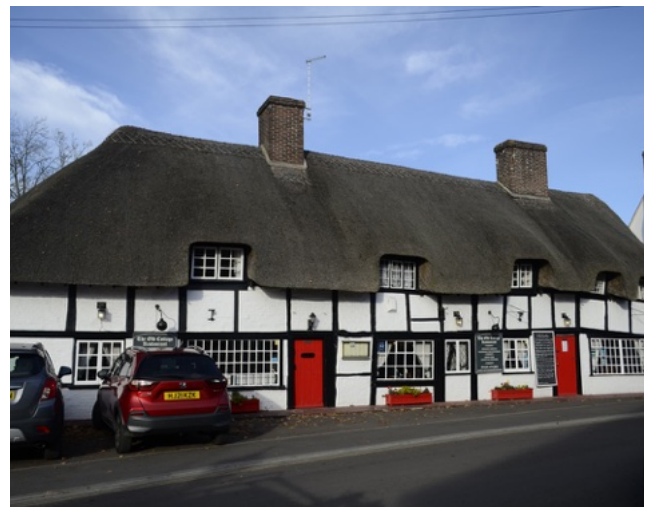
Figure 54: The Old Cottage Restaurant is a Grade II Listed Building, with timber-frame with painted brick and thatch roof.
