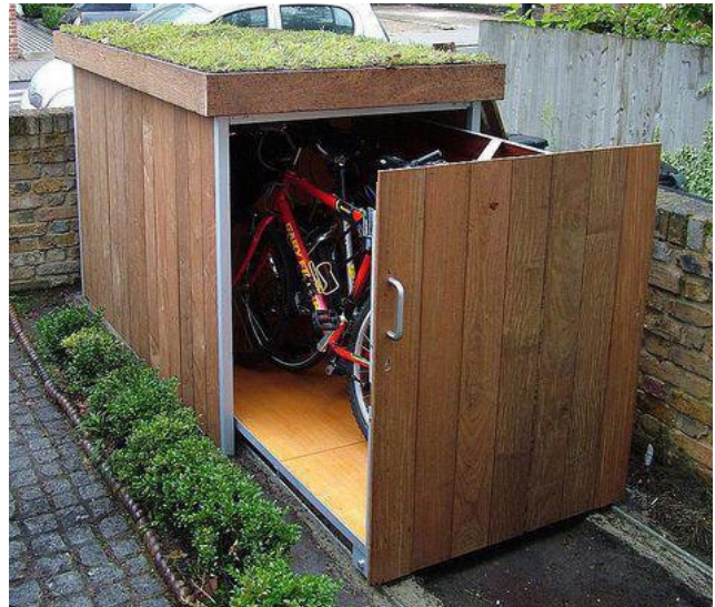
Figure 28: Example of enclosed cycle storage.
