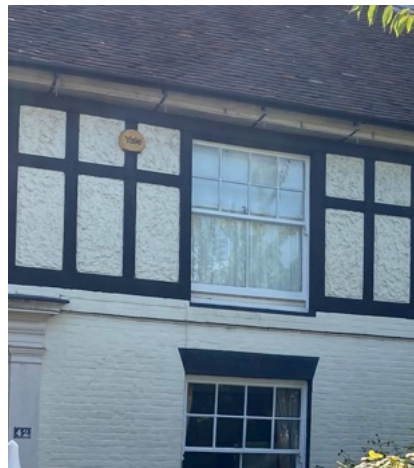
Ground floor in white painted bricks and mixed of roughcast and timber used for second floor
