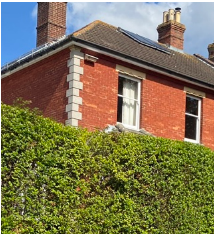
Red bricks building with white cornerstone and inlets stone used as windows details
