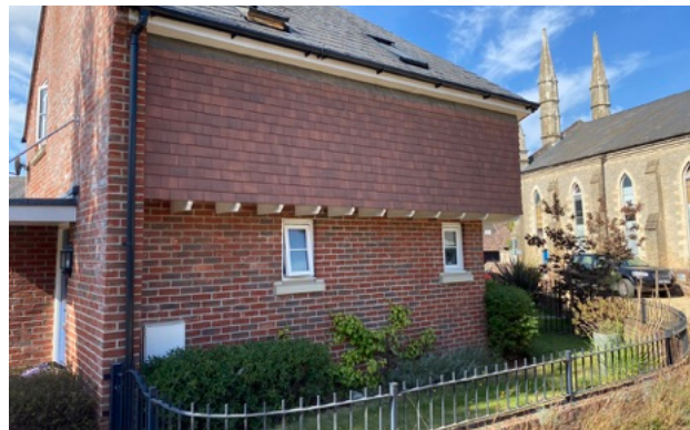
Hung tiles side extension with exposed structure
