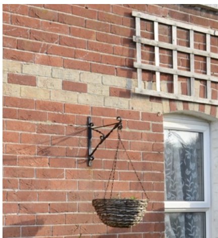
Fascia in buff alternated with red bricks
