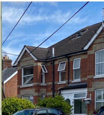
Fascia in buff alternated with red bricks
