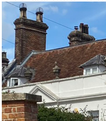
Ground floor in white painted bricks and mixed of roughcast and timber used for second floor
