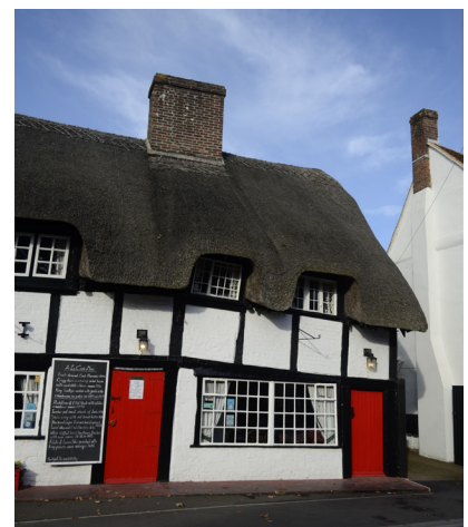
Thatched roof and timbered facade
