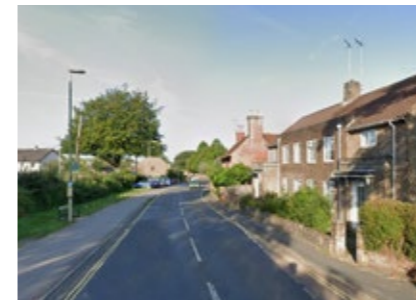
Eastern gateway - Southampton Road
