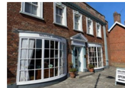
Variety of historic buildings
