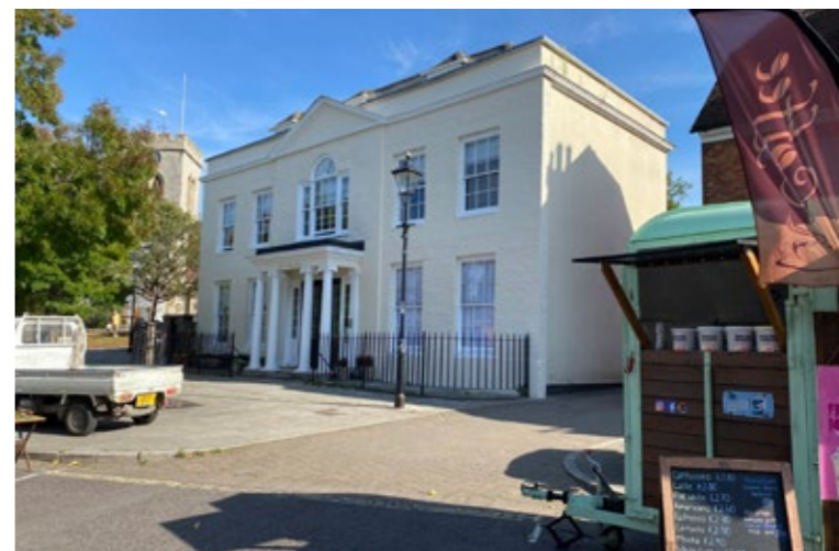
6. Upgrade in paving required
