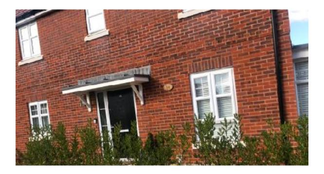
Materials were noticeably cheap; porches & flashings, tiles & slates, window cills, windows & may lead to premature degradation. e.g cills cracking.
