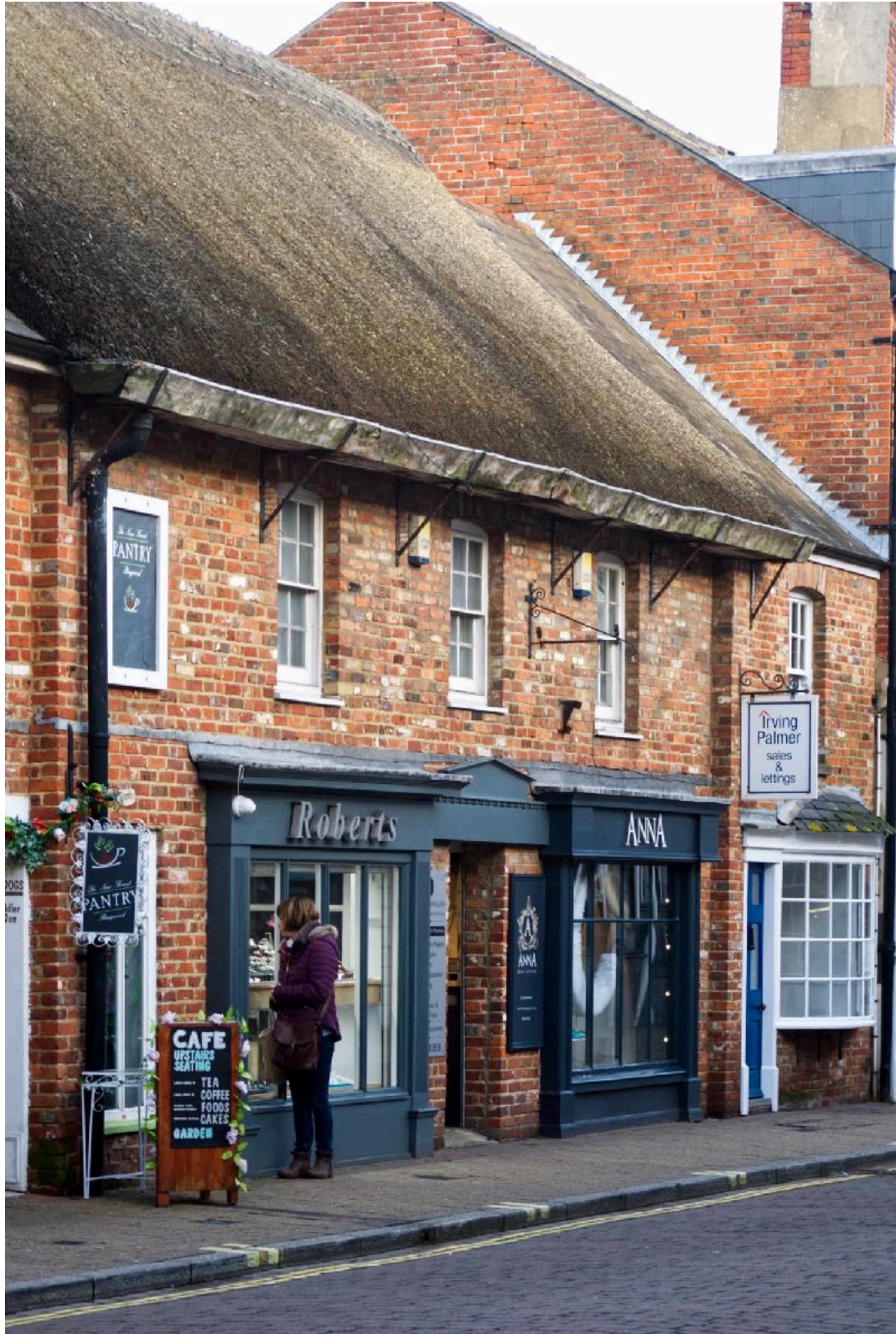
Good recreation of historic building damaged by fire. Roof coverings, windows & timber gutter. (Shopfront in primary shopping area)
