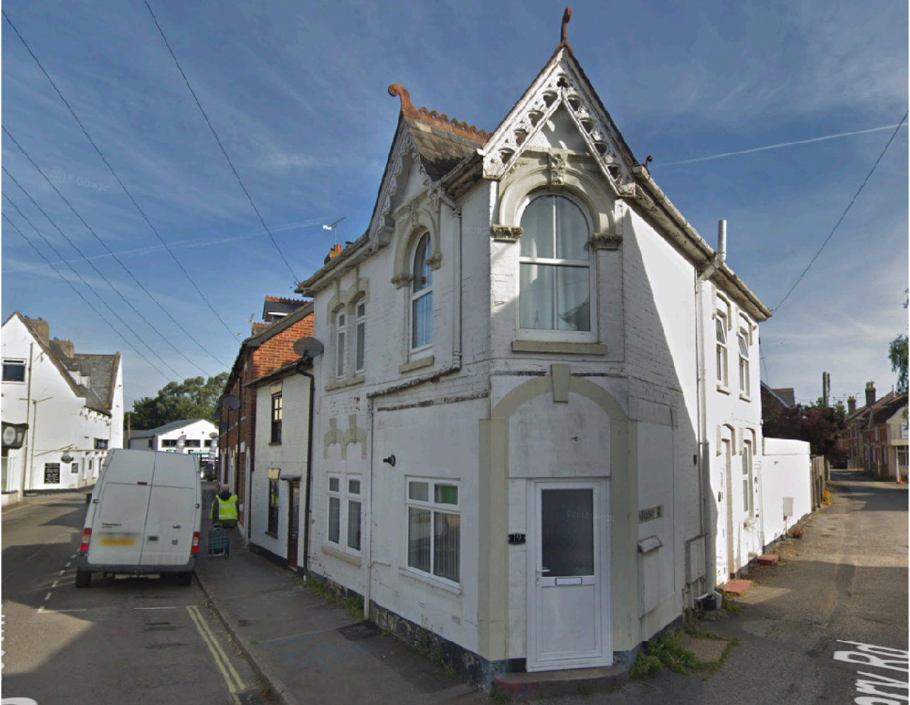
Painted brickwork, door & window alterations, UPVC windows. Roof coverings & ornate barge boards remain.
