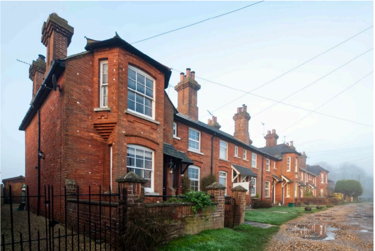
Largely original window patterns, chimneys and roof coverings (some poor windows)
