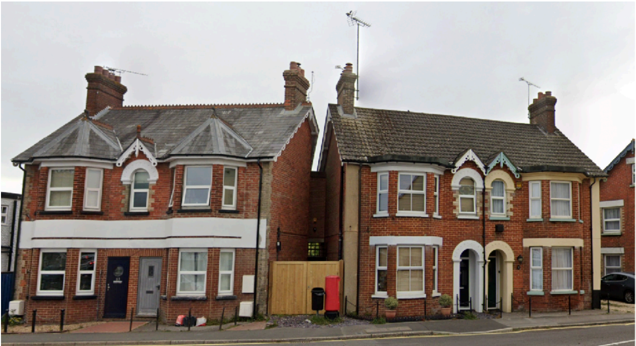
Loss of turrets and slate roof covering on the Right hand pair. Loss of archways on the left. Loss of sash windows to both.
