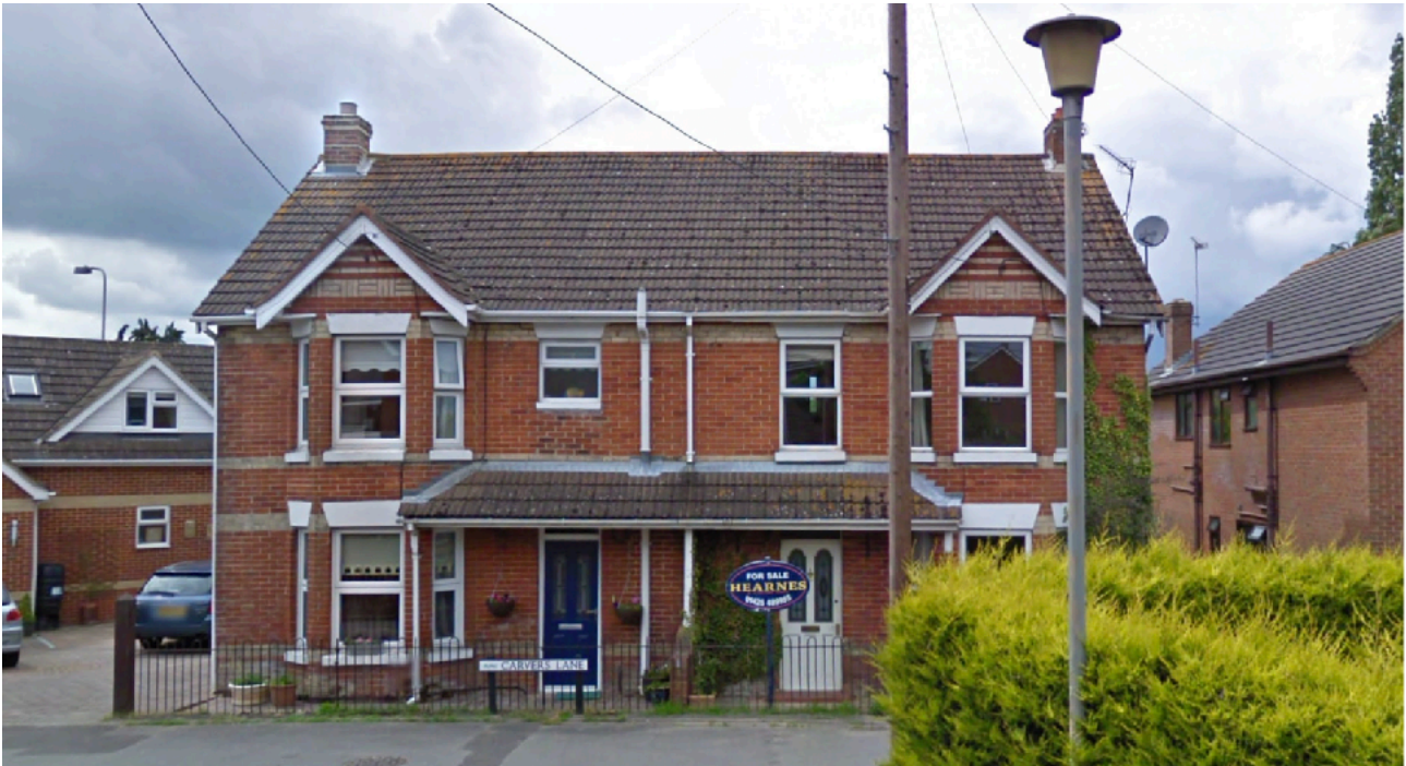
Unsympathetic roof coverings & window alterations. SVP to front elevation.
