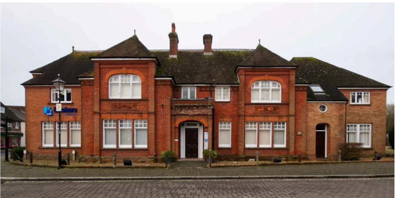
Original openings, brick features & windows
