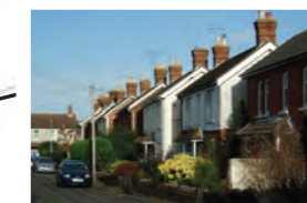
Westbury Road with its turn of the century chimneyed row offers a distinctive skyline both here and at the culmination of Woodford Close behind.
