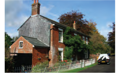
One of the cottages along the route of the old Salisbury Road.
