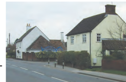
Former Nags Head and one or two rural cottage forms.
