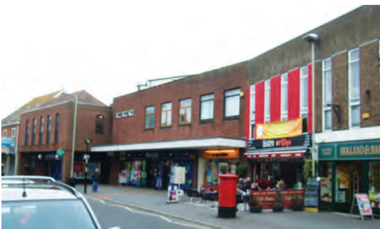
Fig 1.11 The subsequently developed and rather drab run of shops alongside sadly fails to respect the rhythms along the street either through plot division or fenestration pattern (they set up powerful rhythms all of their own). With no roof visible, despite being two-storey, this is equally at odds with the skyline.
