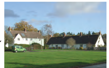
Merryweather Estate the open green and backdrop of garden trees and the forest lands to the east allow utilitarian houses to appear as locally distinct and attractive cottages in a semi-rural setting.
