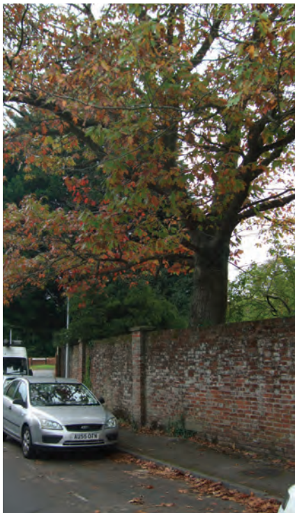
Fig 3.11 The walled garden of Manor House along The Sweep
