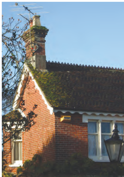
Fig 8.7 Heritage; form and detail. A single late Victorian house pre-dating its similar neighbours by a few years is particularly attractive. It is important that it retains its decorative details, traditional materials and garden setting at the corner of Gypsy Lane.
