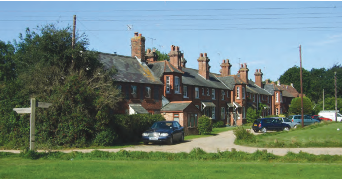
Fig 1.15 Bickerley Terrace – red brick detailing, chimneys and articulated skyline combine with the setting to create a memorable landmark
