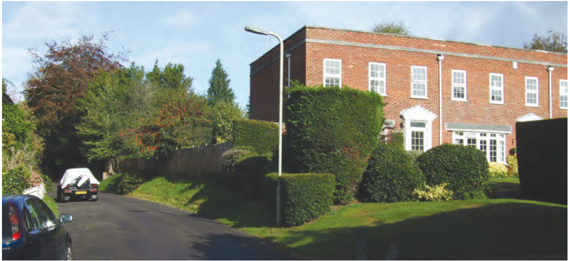
Fig 3.10 Merton Grove from the old Salisbury Road
