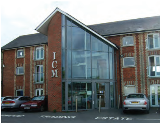
Fig 5.8 A railway related warehouse extended and refurbished to give a new lease of life to this piece of industrial heritage off Castleman Way.
