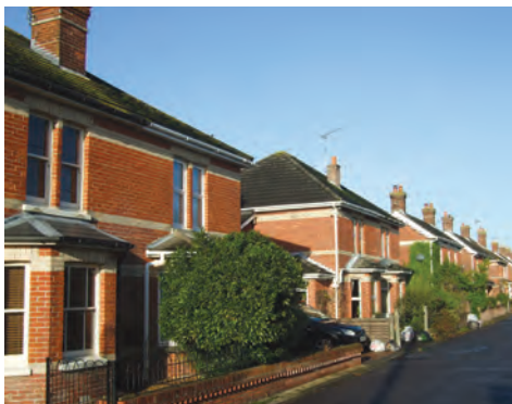
Fig 8.6 Distinctive red and buff brick detail, single storey bays, slate roofs and chimneys at Middleton Road. The front gardens are small but important. Such characteristic elements as these and those listed in paragraph 4.8.5 are worth retaining.
