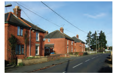
Original red brick semis from early in the twentieth century – unspoiled roof forms, retained chimneys, original window forms and red brickwork are all characteristic
