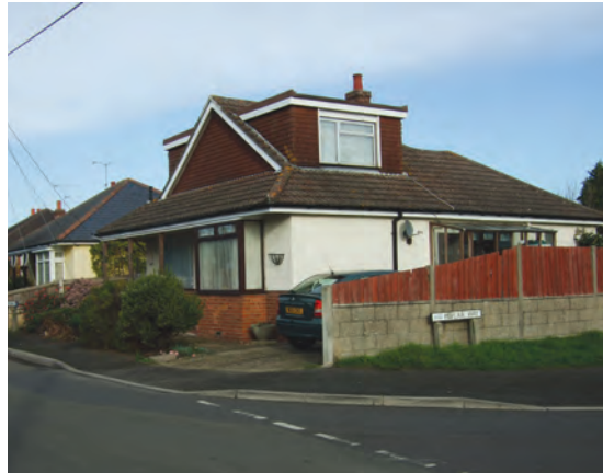
Fig 7.19 A purely functional set of additions
