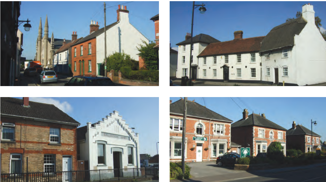
Fig 2.10 Distinctive buildings and harmonious groups along Christchurch Road
