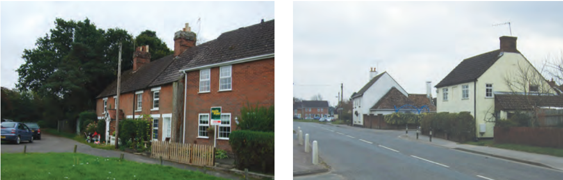
Fig 5.4 Older terraced houses enclose the green and the old Nags Head Inn (now a house) still remains just beyond the north of the triangular green.
