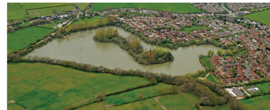
Late C20th estate around Hightown Lake A fairly typical late C20th estate layout, with cul-de-sac arrangement for access.
